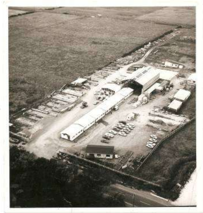
Hydro-scheme housing 1960s-70s: De Geest Construction made 900 houses from workshops in Oamaru and Cromwell
